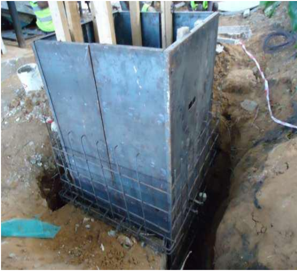
Fixing of manhole reinforcement and formwork
