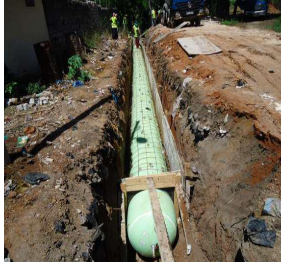
Excavation and setting of pneumatic forms:
