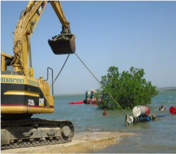
Laying and welding of PLG pipes in sea and mechanical works:
