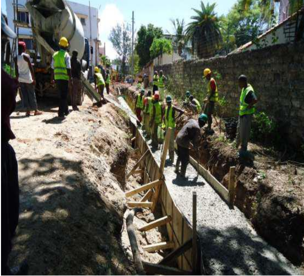
Concrete casting using premix
