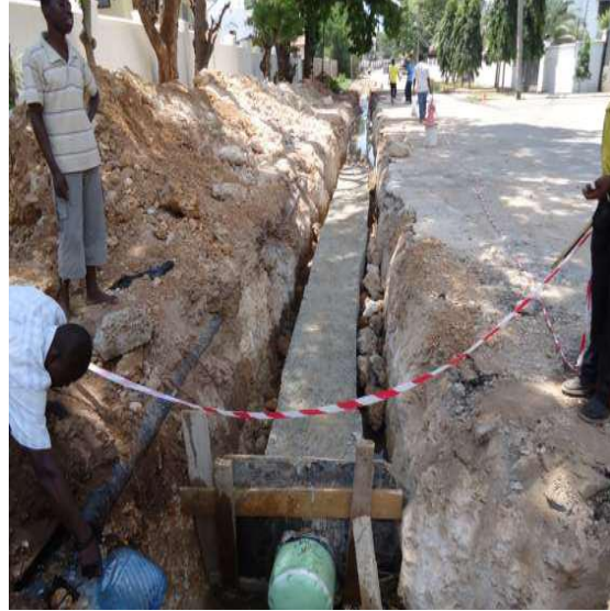
Concrete casting using premix
