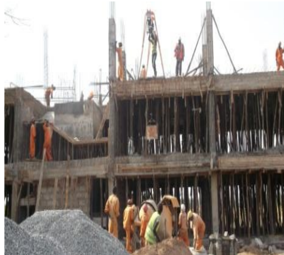
Formwork and scaffolding, reinforcement and concrete works:
