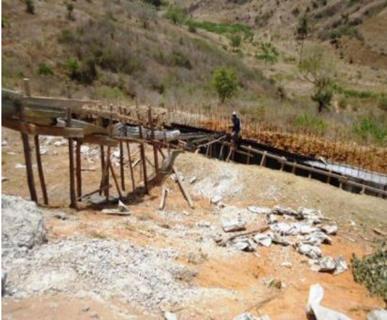
Retaining walls and boundary walls construction
