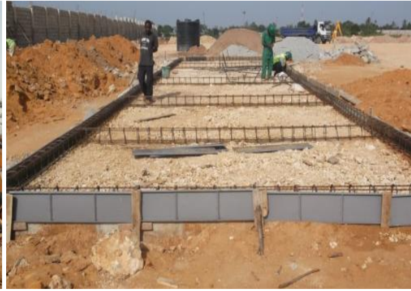
Excavation and setting out and foundation works:
