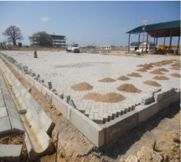
Stabilization, Pavement and drainage works
