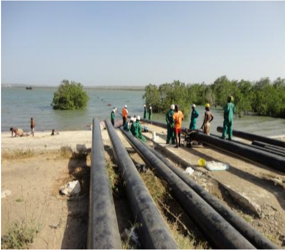
Laying and welding of PLG pipes in sea and mechanical works:
