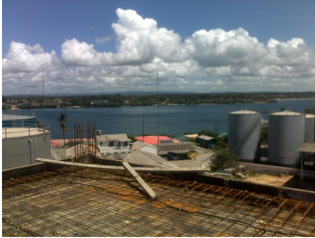
Top slab of office block
