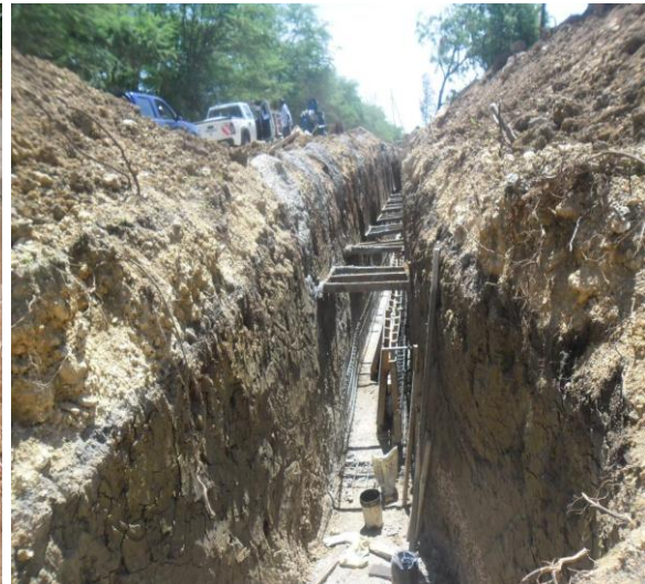
Formwork, reinforcement and concrete works:
