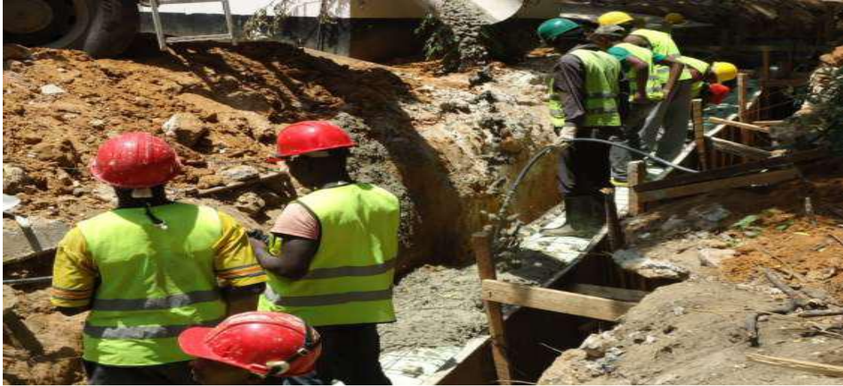
Placing, vibration and curing of concrete in drains
